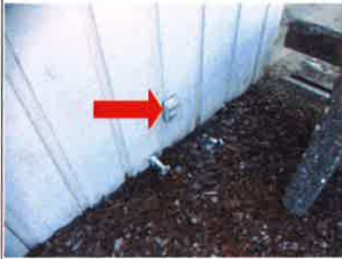
Receptacle at north side did Not function.
