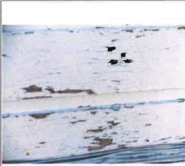
Example of some cladding needing treatment due to weathering.
