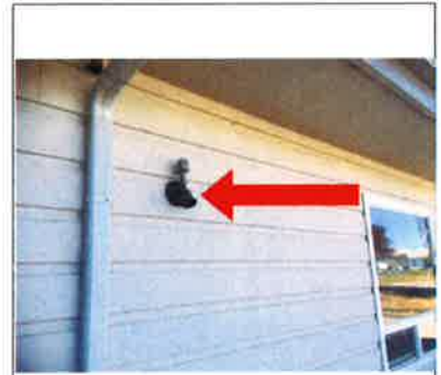
Open light socket on north side.
