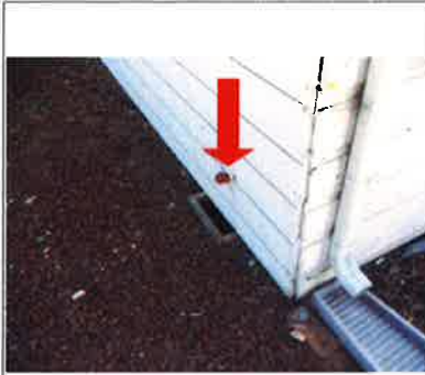
Receptacle at N-W corner did Not function.
