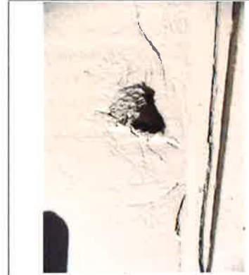
Example of holes from knots.
