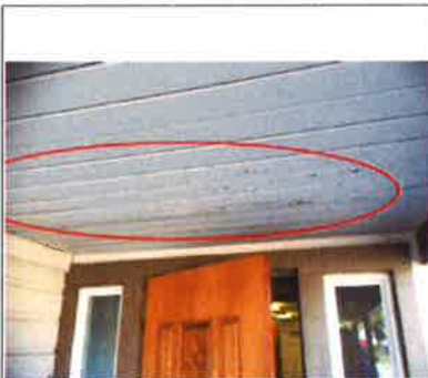
Soffit is decayed above front porch towards the front door.
