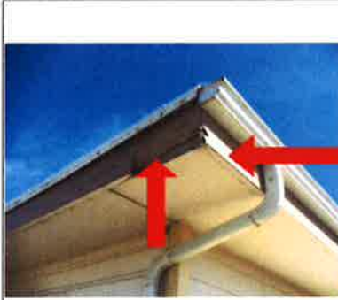
Fascia is damaged at the S-W corner.
