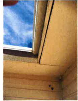
Fascia is warped and has created a gap that can allow bats, insects or rodents to enter the soffit area at corner inside the propane tank fenced area.
