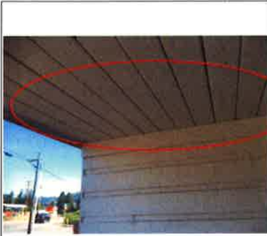
Soffit is also decayed at the north end of front porch.
