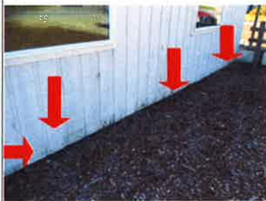
The bottom of siding is decayed all along the north side left of front porch, likely from being in contact with soil.
