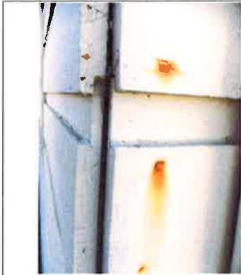
Example of some fasteners having corrosion.
