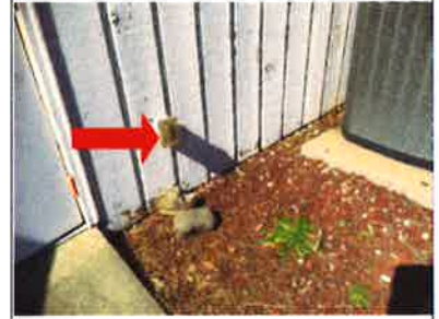
Receptacle at east side did Not function.
