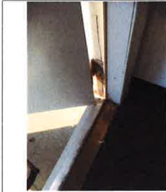
Easterly of the two rear doors is also weathered and has water-stains on threshold.
