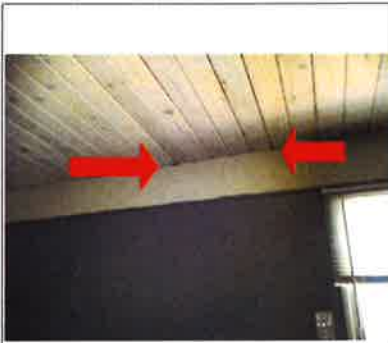
Decayed wood where ceiling meets south wall inside S-E Corner Gray Room.
