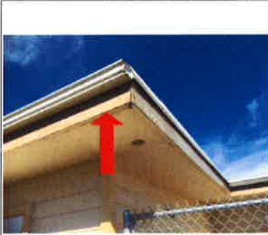
Fascia has decay at the corner near the propane tank.
