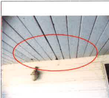
Soffit is decayed above front porch near the exterior light fixture.
