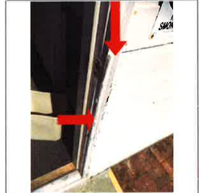
Trim has decay on easterly of the two south rear doors.
