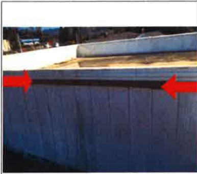
Trim is decayed at the Parapet Wall above the front porch.
