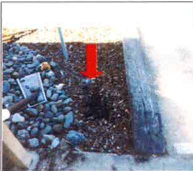
Hose Bib at corner of front porch leaks.
